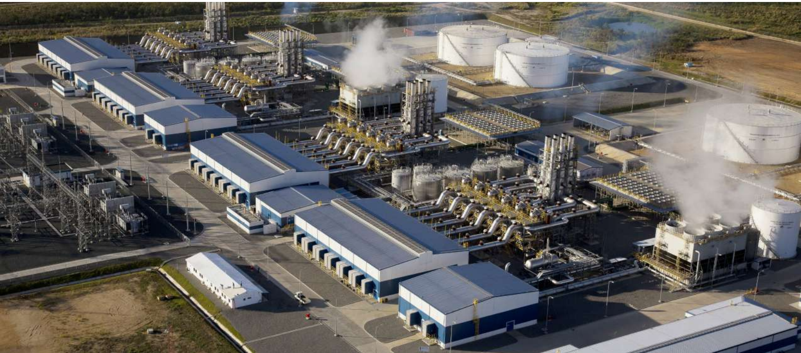
In the Dominican Republic, the Quisqueya 1 power plant has been converted to accept natural gas instead of heavy fuel oil. It is expected to cut Pueblo Viejo's CO 2 emissions by 260,000 tonnes per year.
