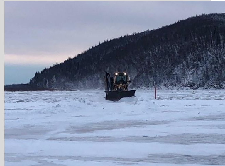
Clearing the ice road near Aniak, AK, February 2020
