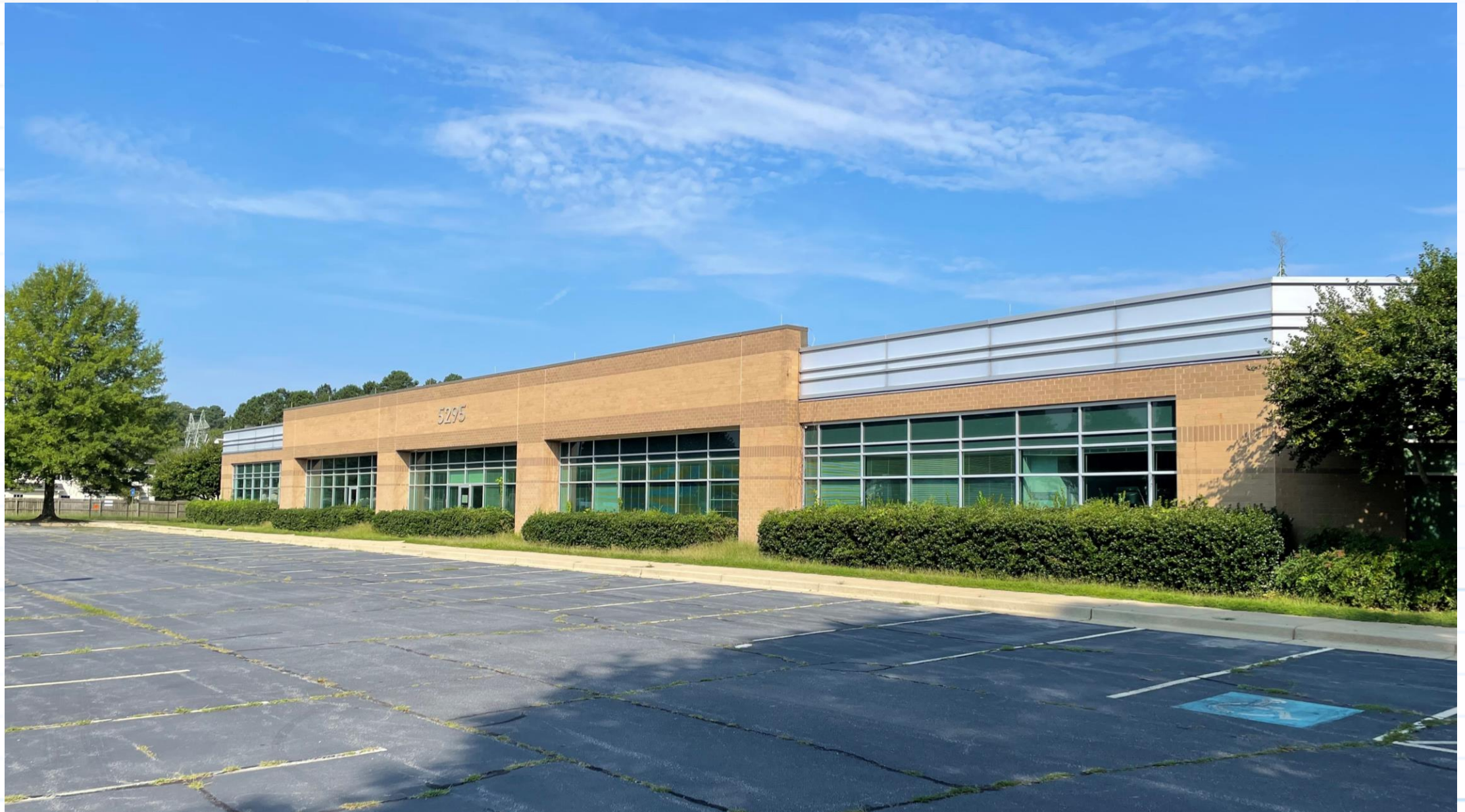
NORCROSS DATA CENTER - ATLANTA
