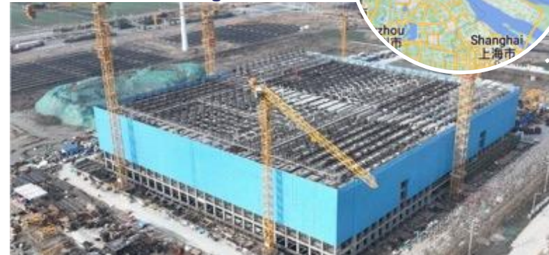
Site Construction Progress
