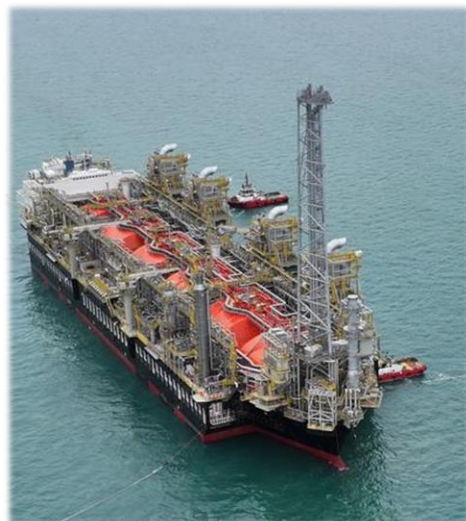
FLNG Gimi (ready for operations) – MKI (2.7mtpa) 1)
