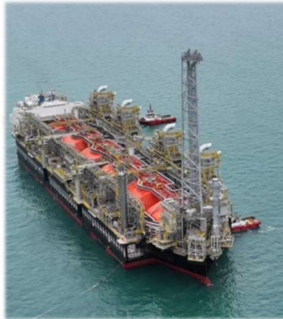
FLNG Gimi (ready for operations) - MKI (2.7mtpa 1 )
