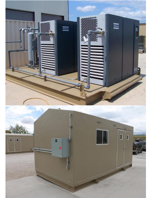
Utility air package used to replace gas pneumatic devices that lower customers GHG emissions, assisting with customer net-zero goals
