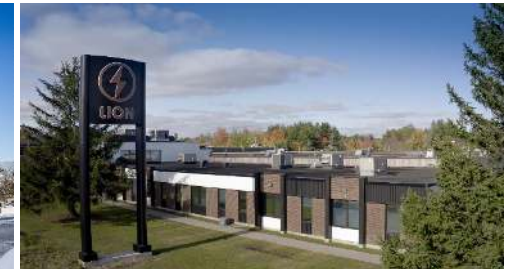
MANUFACTURING FACILITY IN ST-JEROME (MONTREAL), QC
