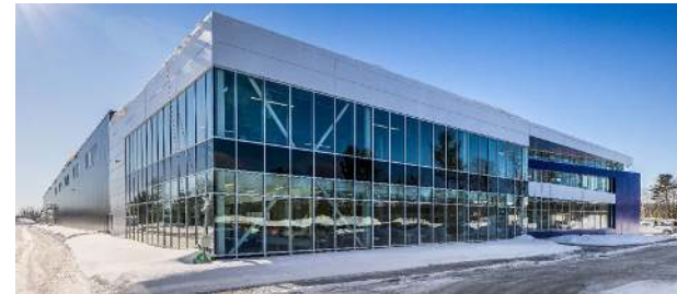
BATTERY PLANT IN MIRABEL, QC
