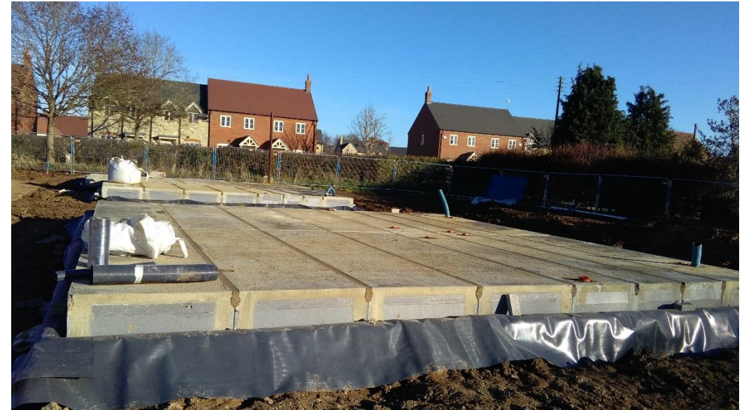
Off-site foundation system trial
