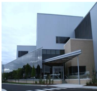
Manufacturing Facility Danbury, CT
