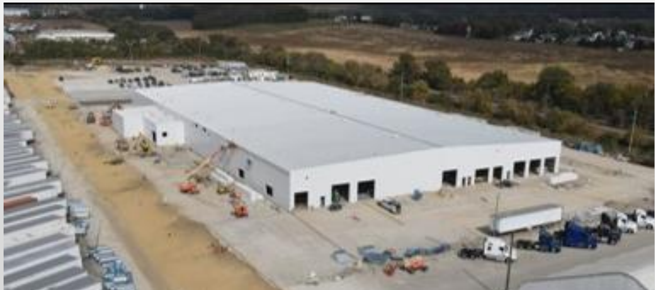
Kenworth New Test Building, Chillicothe, OH
