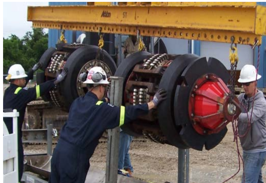
36-inch Magnetic Flux Axial Flow Detection In-Line Inspection tool being loaded into Line X
