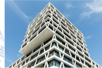
Uponor heating & cooling solutions - winner of Diamond & Gold awards from German Sustainable Building Council (DGNB): 50Hertz headquarters, Berlin, Germany
