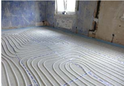
Radiant heating and cooling
