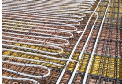
Thermally active slabs
