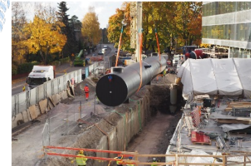
Weholite stormwater tank to attenuate runoffs at the new Children's Hospital: Helsinki, Finland
