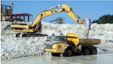
On-site Mining / Excavation
