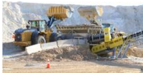
Conveyer Belt to On-site Wet Plant
