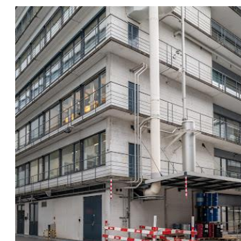
Site for planned device pilot facility in Basel
