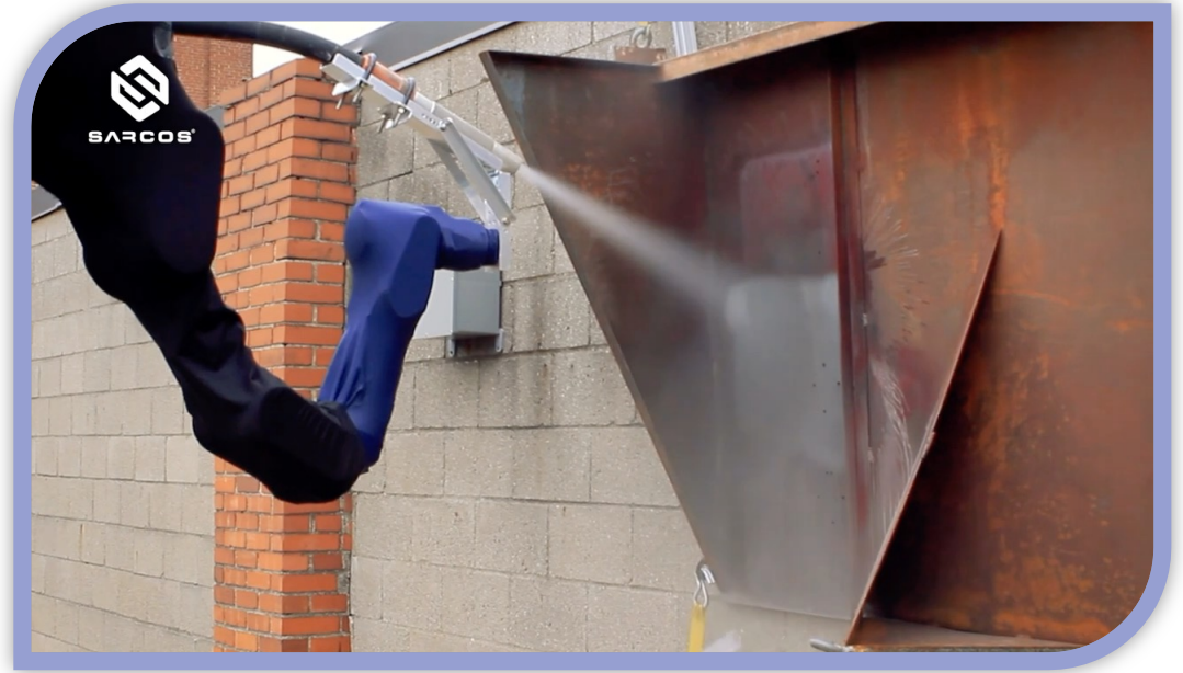
Media blasting to remove paint & rust
