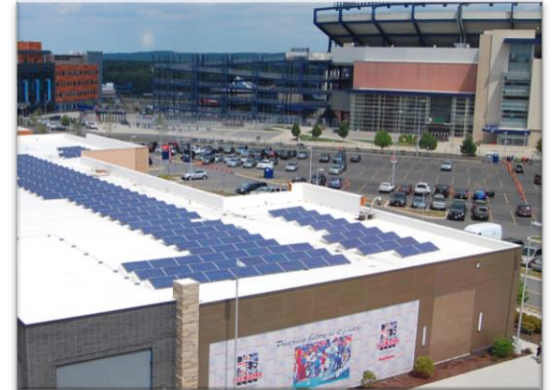
New England Patriots Complex MEP, Telecom & Commissioning Services Foxborough, MA
