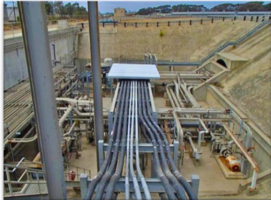
Poseldon Desalination Project Design & Construction Support Services Carlsbad, CA
