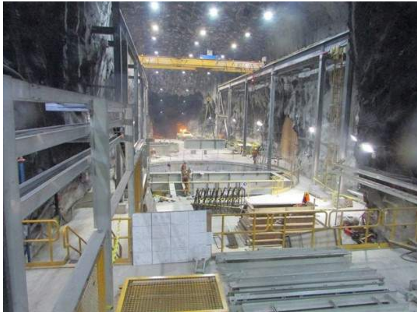
Freeport Underground Mine, sheave deck installation, Indonesia
