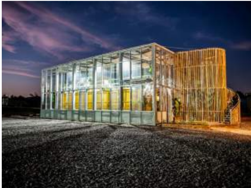
Organica Water Reclamation Demonstration Plant, Verulam, South Africa
