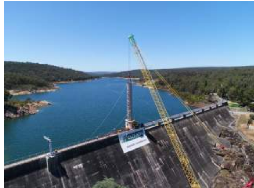
Mundaring Weir outlet works upgrade, Mundaring, Western Australia
