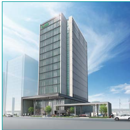
Shimane Bank's Head Office
