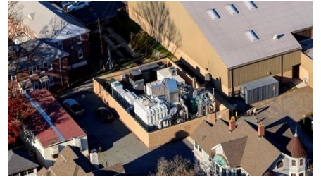
FuelCell Providing On-Site Power Generation
