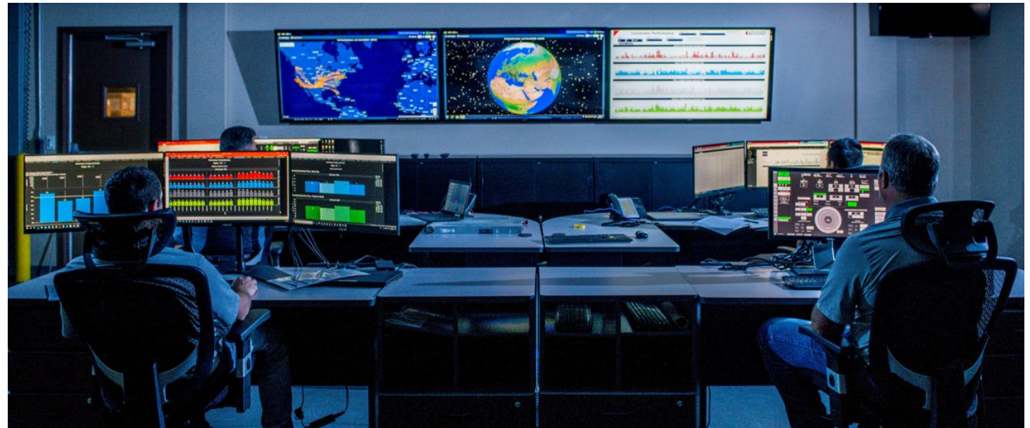
Ensign's EDGE & APM Operations Centre Remotely monitoring our global Edge operations in real-time
