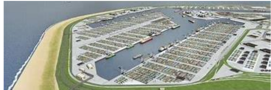
Port of Rotterdam Maasvlakte II expansion
