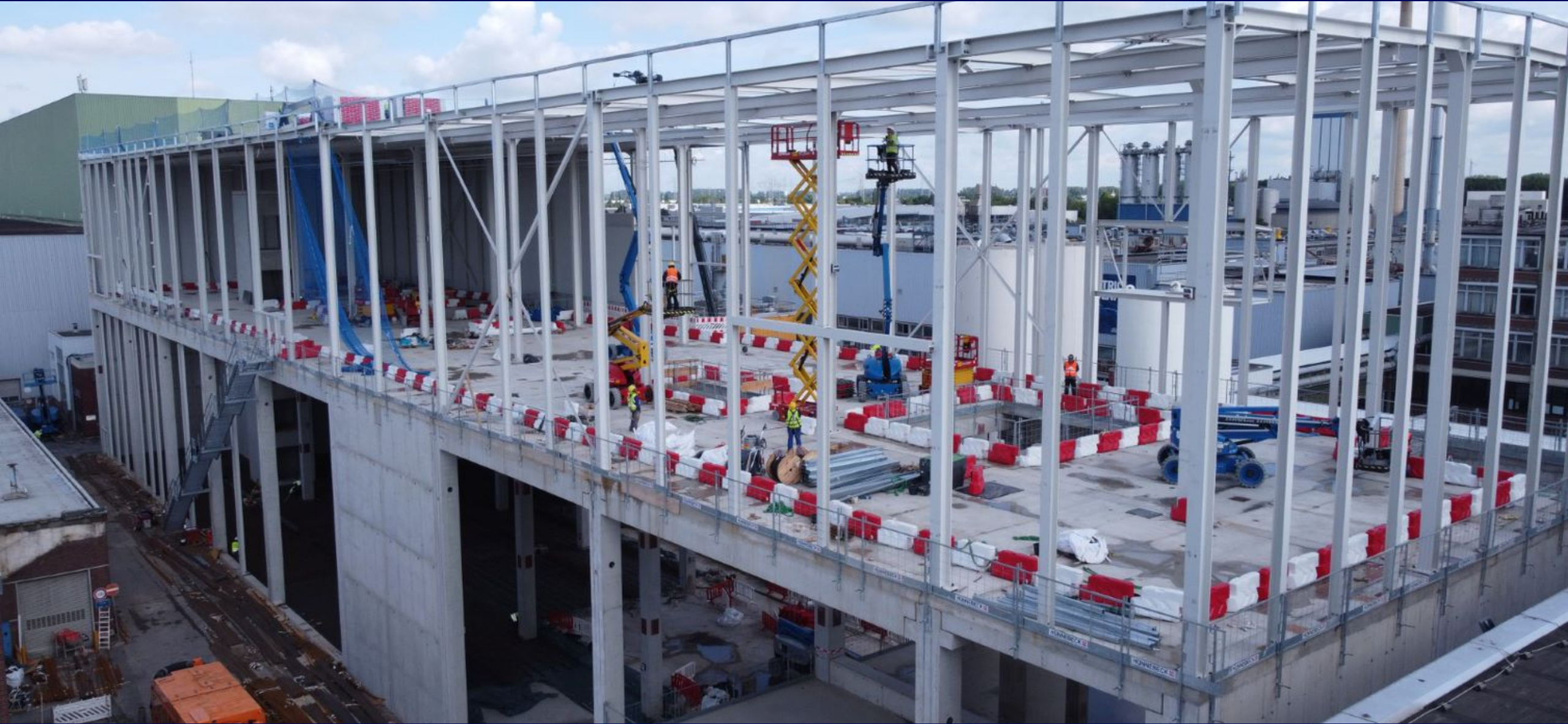
Cologne Electrification Center Construction
