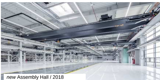
new Assembly Hall / 2018
