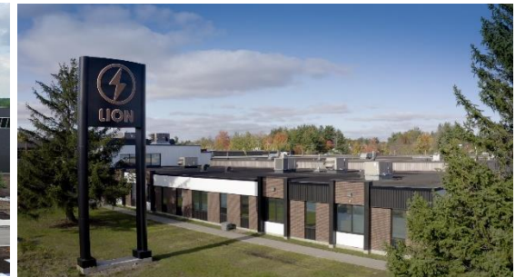
MANUFACTURING FACILITY IN ST-JEROME (MONTREAL), QC
