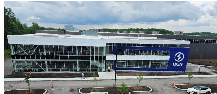
BATTERY PLANT IN MIRABEL, QC
