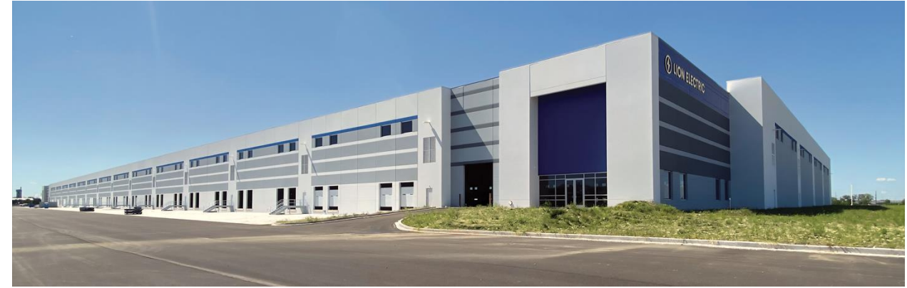
MANUFACTURING FACILITY IN JOLIET, IL
