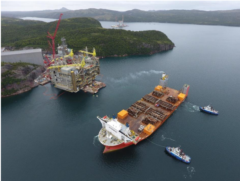
Hebron Utilities and Process Module (UPM) Offloading
