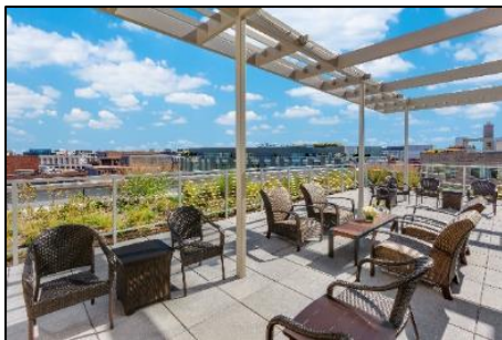
Green roof at Hersha's Hilton Garden Inn M Street, DC, a LEED Silver hotel
