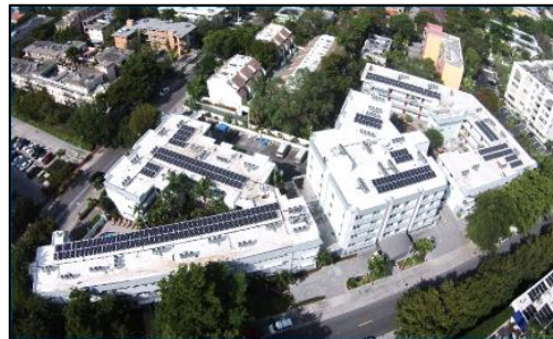
336-panel solar photovoltaic system on the roof of Residence Inn Coconut Grove, FL
