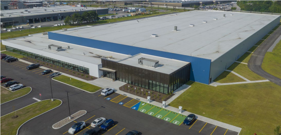
WAREHOUSE: Complete and Certificate of Occupancy
