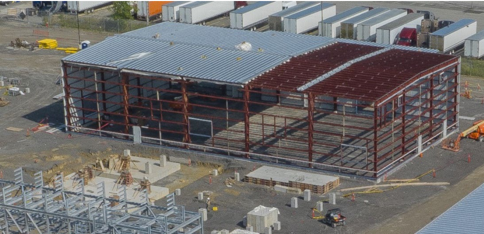
FINISHED PRODUCTS AREA: Advanced Steel Erection
