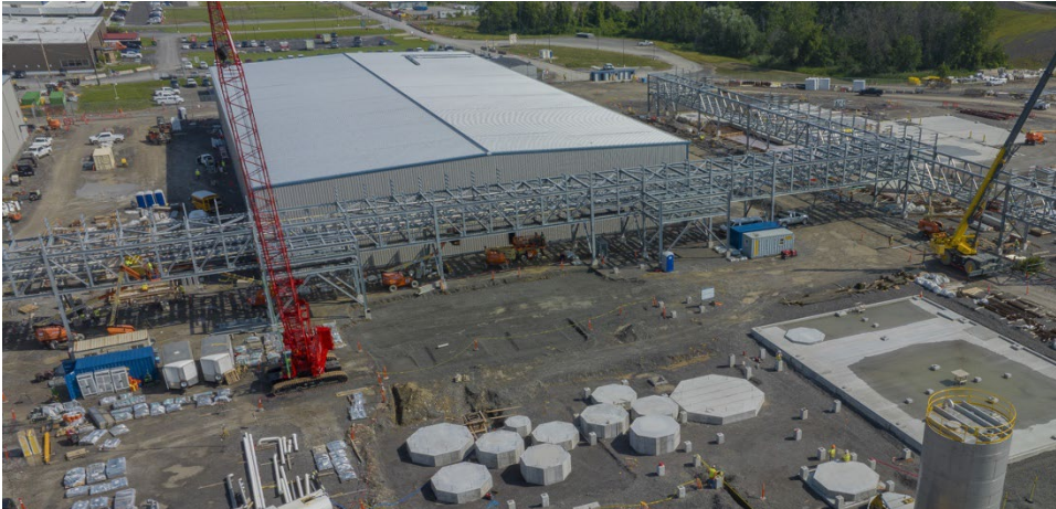
MAIN PIPE RACKING: Advanced installation
