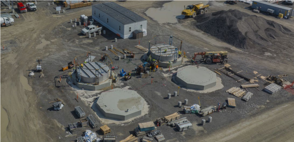
CONCRETE TANK FOUNDATIONS: Largely Complete
