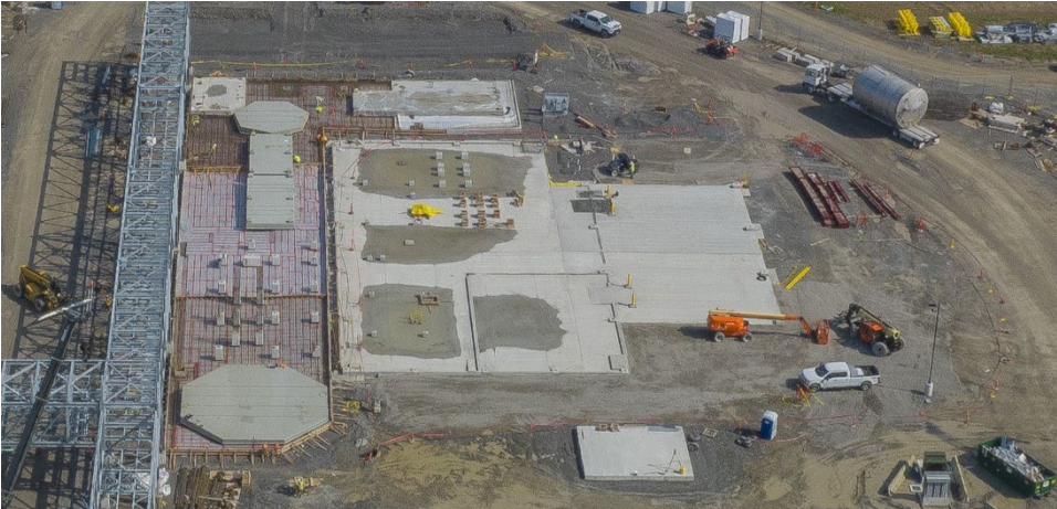
LEACHING: Building Steel Underway
