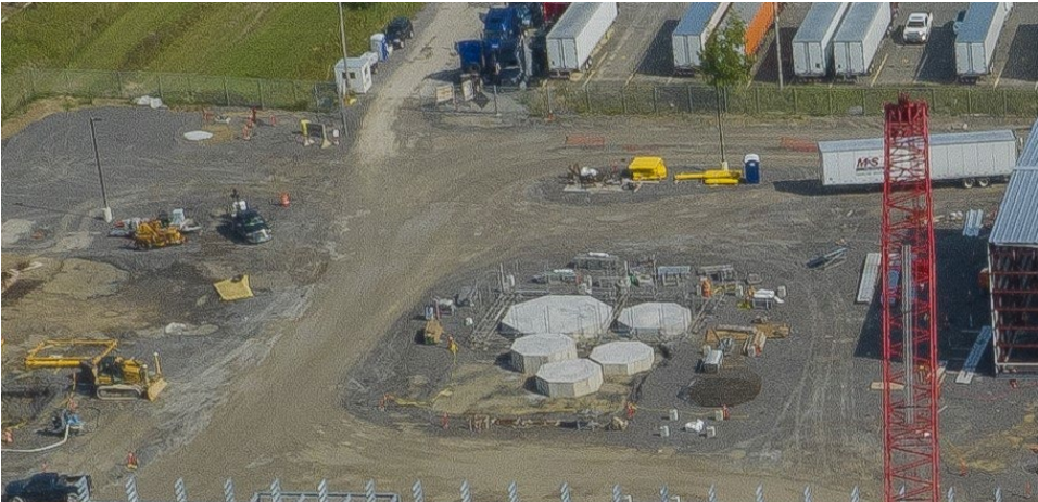
LITHIUM: Building Foundation Underway
