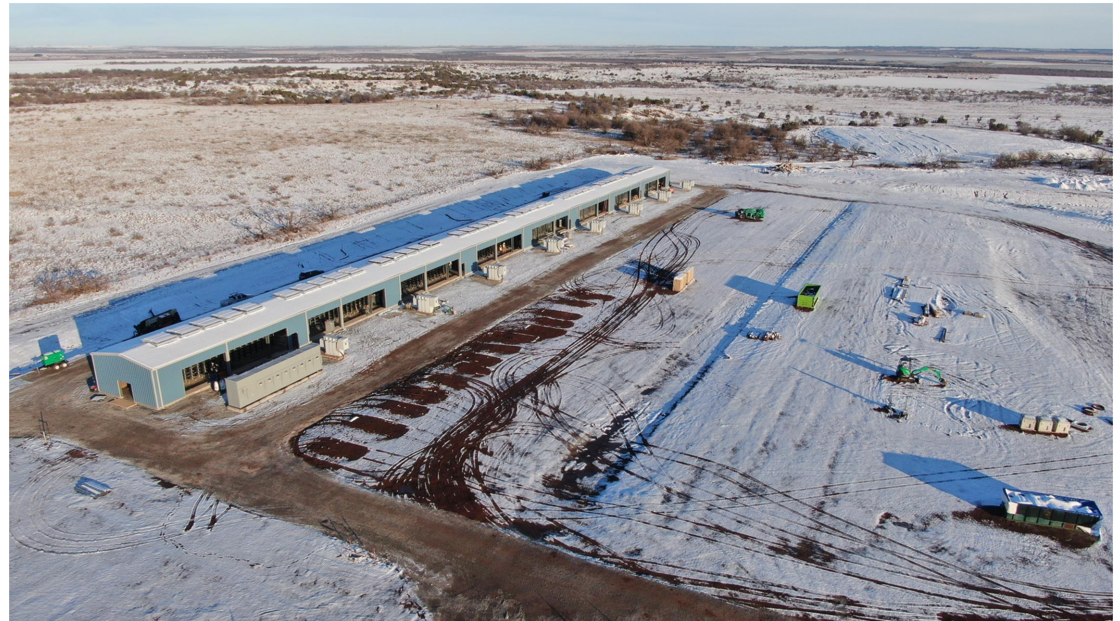
Childress (January 2023) - aerial view of the first 20MW data center building
